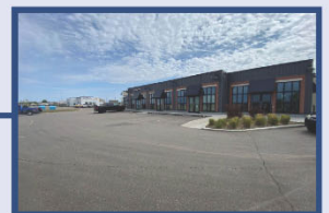
Highway commercial and retail development
